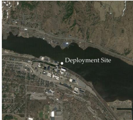
Figure 1. Aerial view of MTU Site
